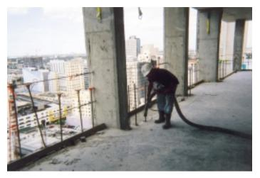
A lot of repositioning from one block cell to the next occurred when crews had to place concrete through 4-inch knock-outs in the floor above the blocks.
