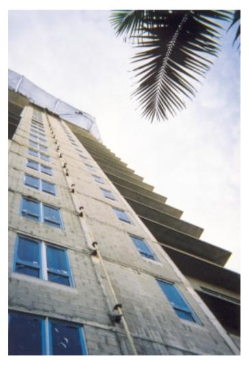
A Putzmeister TK 40 was required to pump concrete up through 270-ft of pipe extending vertically against the side of the building and then through another 300-ft of hose placed horizontally on each floor.
