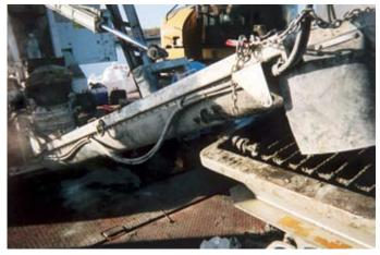
Tremie pours were performed, employing a high strength 7,000-psi concrete and the efficiency of a Putzmeister trailer pump.
