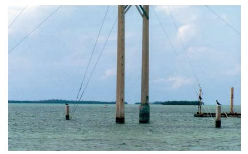
A million dollar contract by Keys Energy Services required Underwater Engineering Services to seal minor cracks and replace over 100 corroded power poles found in the waters of Key West.
