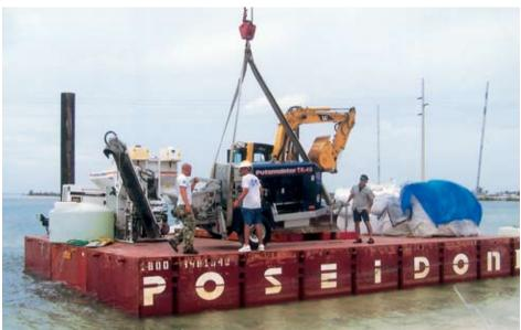
A crane lifts and extends a Thom-Katt TK 40 trailer-mounted concrete pump over water, positioning it a mere six inches from the barge's edge to maximize space. The pump was supplied by Quality Concrete Pumping of Coral Springs, FL for continuous use over a ten week period.
